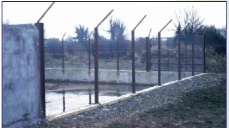
All slurry tanks should be adequately fenced.
